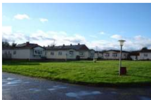
Poplars Park mobile home site
