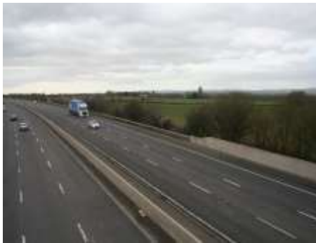
M5 from bridge on A4137
