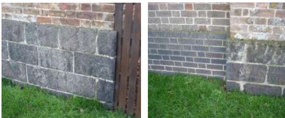
Original and conventional black bricks at Kingston House
